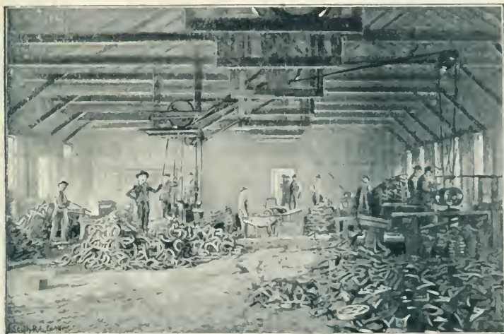
FORGE ROOMS, AGRICULTURAL WORKS.
