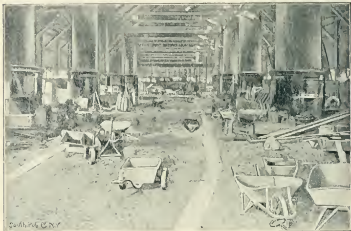
PUDDLING FURNACES, LOOKOUT ROLLING MILL.
